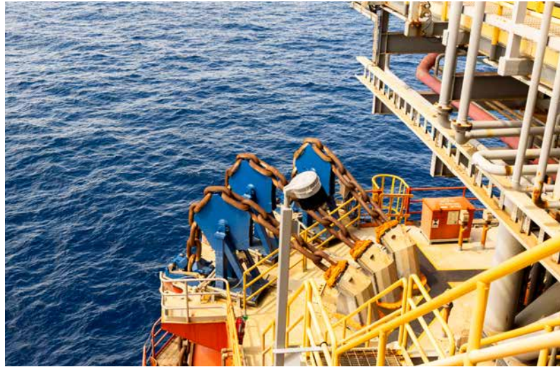
Mooring anchor chains on the Who Dat FPS, Gulf of America, USA
