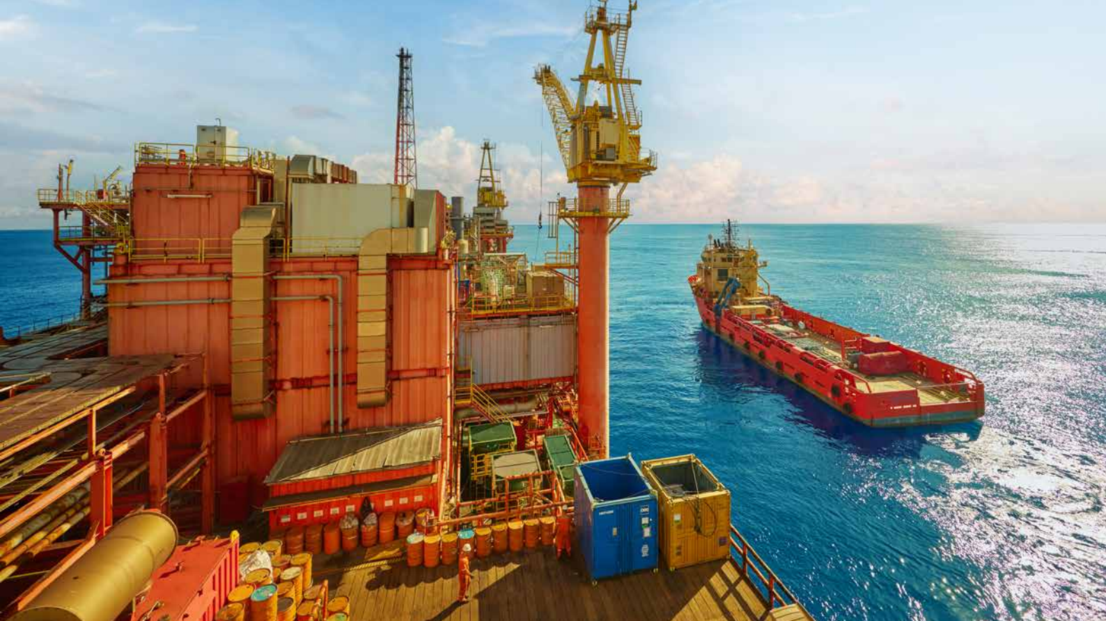
Baúna FPSO (left) and supply vessel (right)
