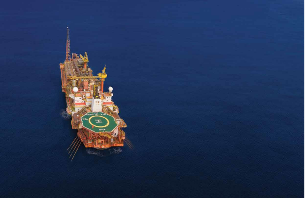
Baúna FPSO, Santos Basin, Brazil
