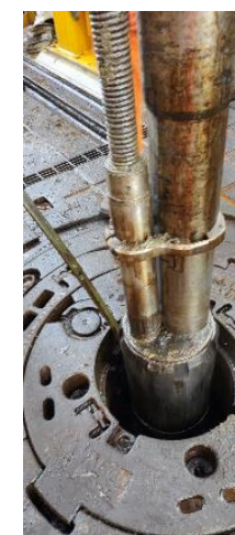
Electrical Submersible Pump (ESP)
