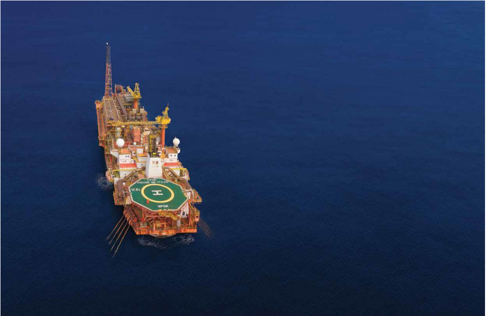
Baúna FPSO, Santos Basin, Brazil
