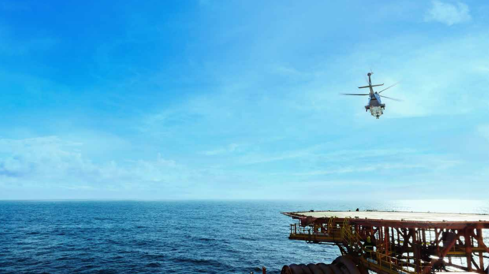
FPSO transport helicopter taking off from Baúna FPSO, Santos Basin, Brazil.
