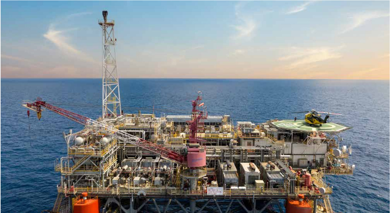
Topside facilities, Who Dat FPS, Gulf of America, USA
