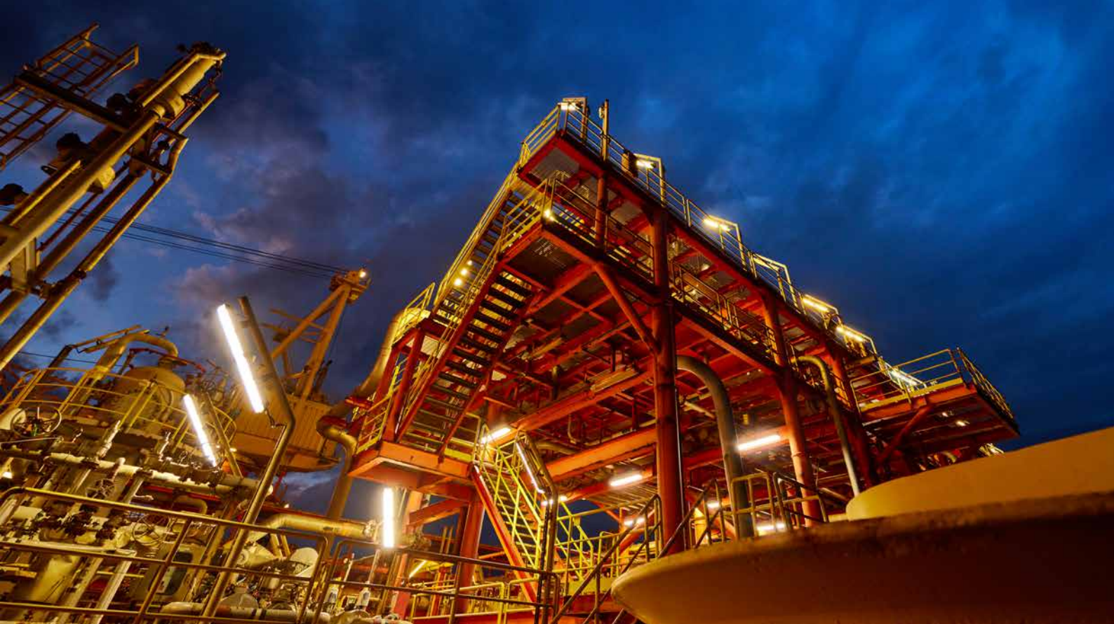
Baúna FPSO, Santos Basin, Brazil.
